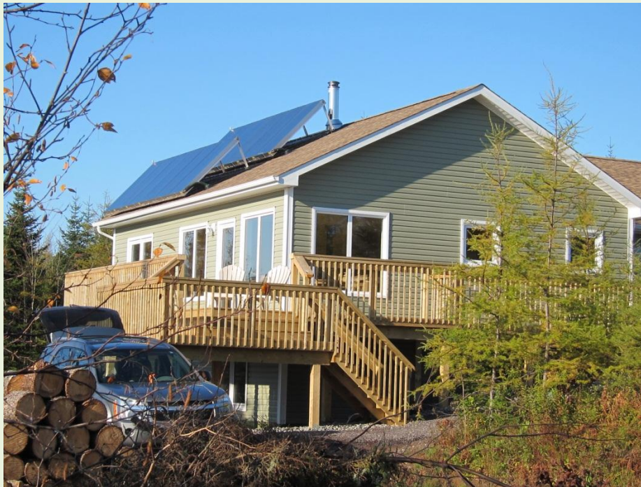
2 * 6 * KA88/2002 (two rows) for solar domestic hot water and space heating
