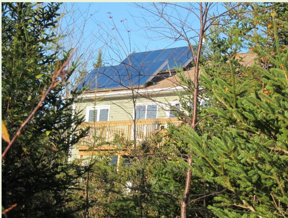
2 * 6 * KA88/2002 (two rows) for solar domestic hot water and space heating
